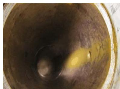
Offshore water suction line, over 70% blocked, required 5 soakings of 20% solution for complete removal.
